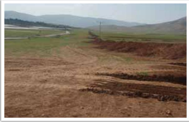
Trenches (or ditches): are dug across flat land or along the side of a road to prevent vehicles from going around a closure obstacle on the road.
