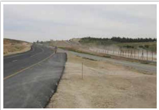
Road Barriers: may be composed of a fence or a concrete barrier running along the side of a road. To be classified as a road barrier, this type of infrastructure should be at least 100 metres long and obstruct free passage of people, vehicles or livestock, onto, off or across the road.
