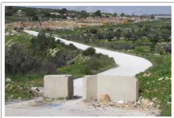
**Roadblocks:** are constructed from one or more concrete blocks of about one cubic meter and, like earthmounds, are used to prevent vehicle access to land or roads. In all other respects, they are the same as earthmounds.
