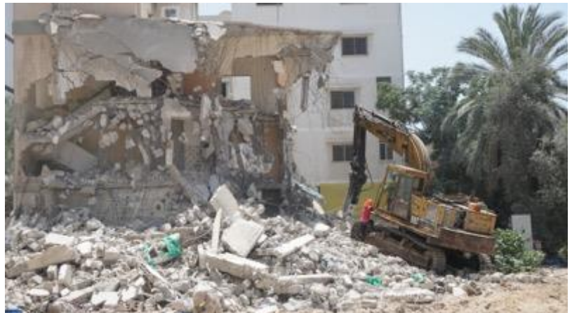
Egyptian-donated building equipment to support Gaza rubble removal. June 2021 © OCHA
