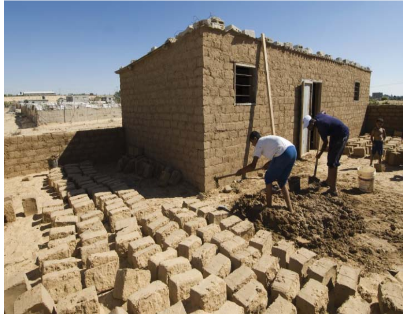
House constructed with mud bricks, Rafah. June 2009.
