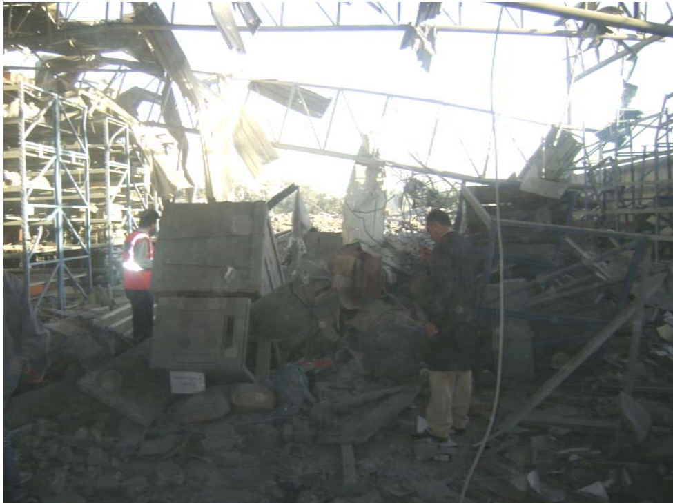
Paltel Group's main warehouse
