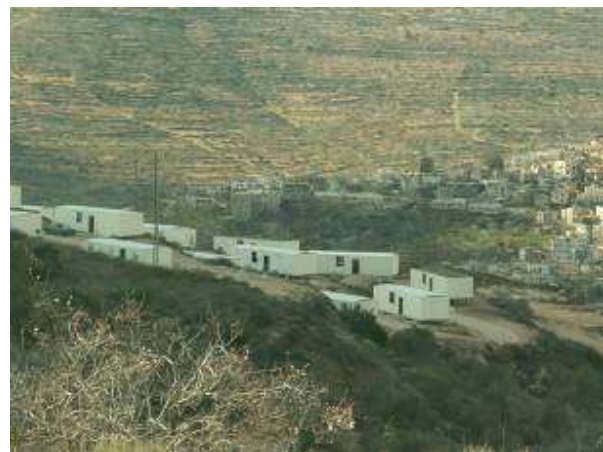
Construction East of the Fence, Eli, 11.2.08
