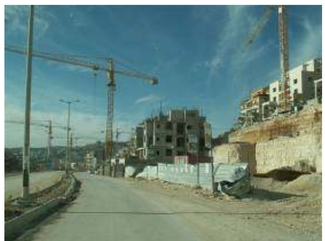
Construction in Har Homa, East Jerusalem
