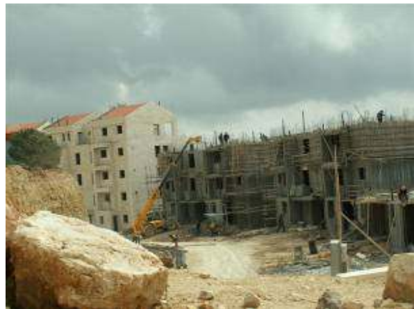
Construction West of the Fence, Giva't Ze'ev, 5.3.08
