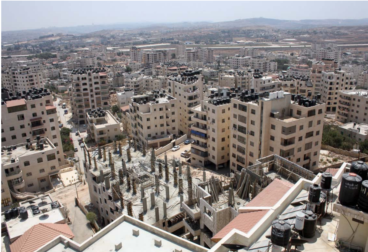
Construction boom in Kufra Aqab. August 2010, Al-Haq©.
