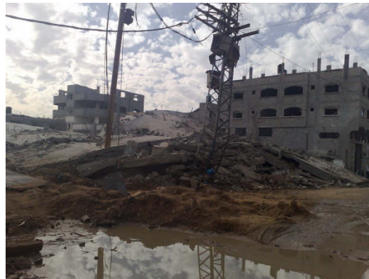
Damages in Beit Hanoun, picture supplied by PHG
