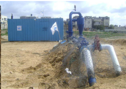
Khadeeja well after repairs, picture provided by CMWU
