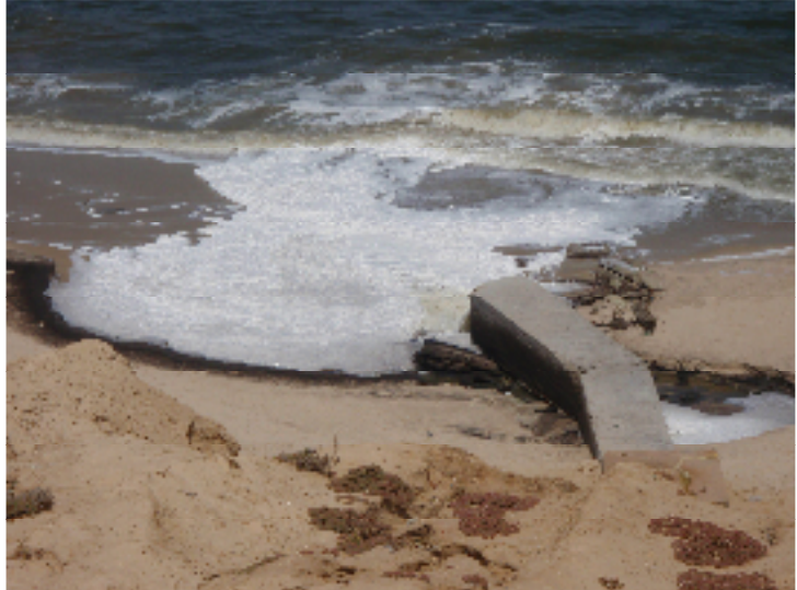
Sewage outflow from Gaza WWTP
