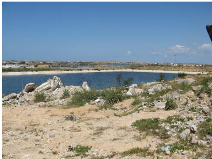
Beit Lahia Wastewater Treatment Plant, picture provided by Graham Henderson
