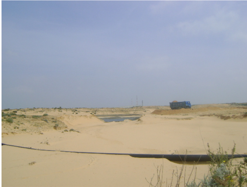
Figure 9 Opening at the embankment of the temporary disposal ponds (Photograph by the CMWU on 2 nd April 2009)
