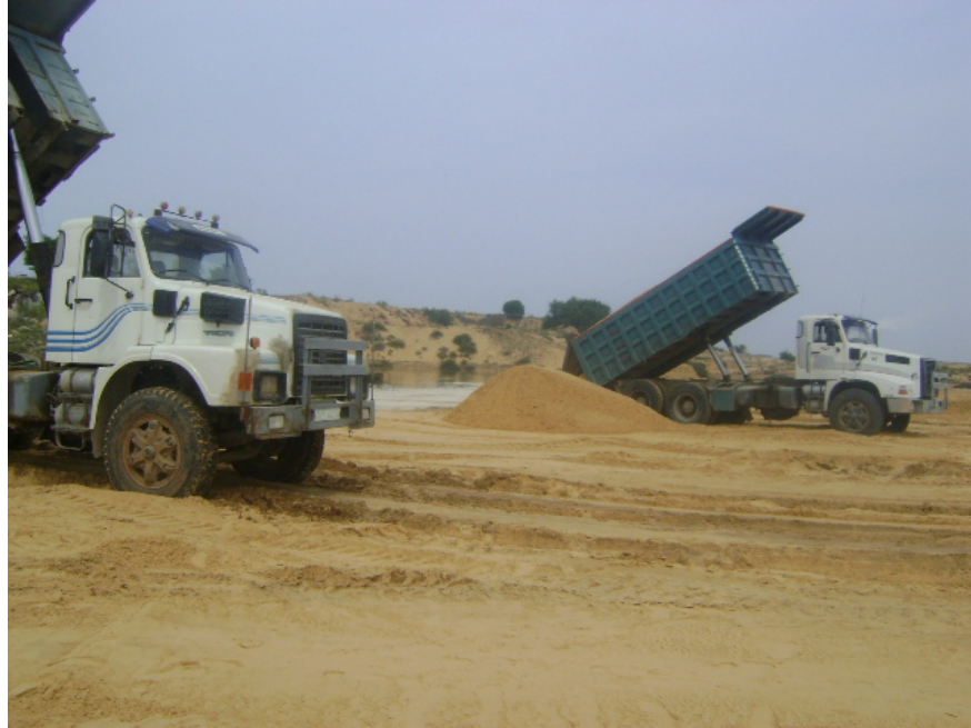
Figure 6 Sand being dropped by the CMWU contractor at the stationery leading edge of the escaped wastewater (Photograph by CMWU, received by the WASH Cluster Team on 6 th April 2009)
