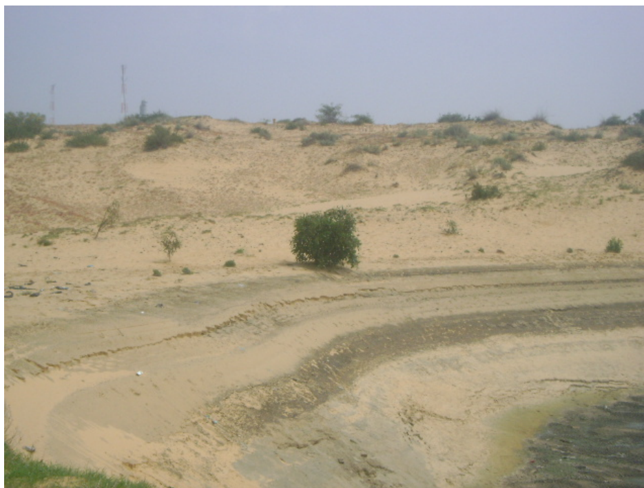
Figure 15 A view of one of the two temporary disposal ponds (where the collapse occurred) (Photograph by the CMWU on 2 nd April 2009)
