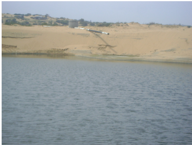
Figure 14 Inlet pipe to the northern-eastern ponds (temporary disposal ponds) (Photograph by the CMWU on 2 nd April 2009)
