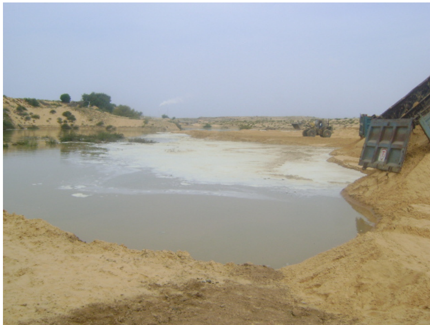
Figure 7 Sand being dropped and positioned by the CMWU contractor at the stationery leading edge of the escaped wastewater (Photograph by CMWU, received by WASH Cluster Team on 6 th April 2009)
