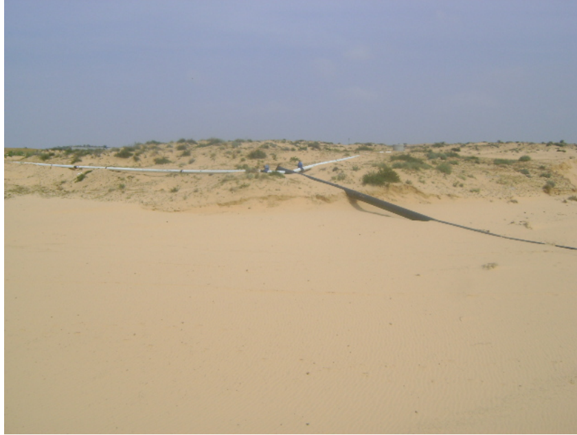
Figure 13 Existing distribution pipes from the BLWWTP to the two temporary disposal ponds. (Photograph by the CMWU on 2 nd April 2009)
