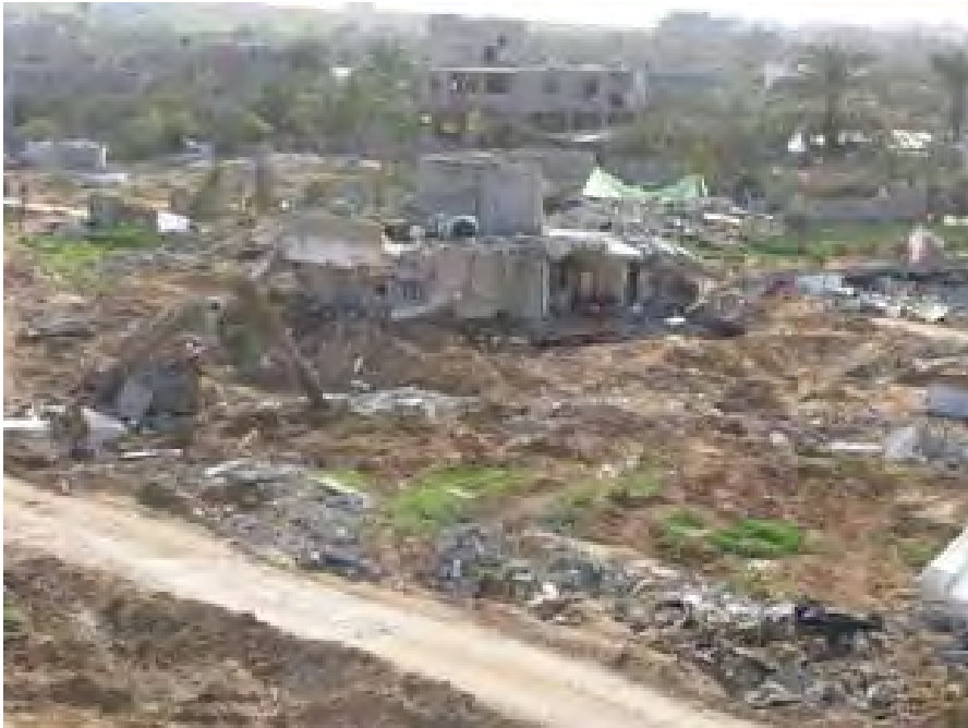
Damages in private properties and roads
