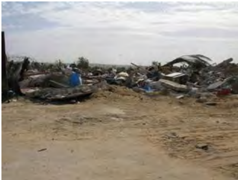
Damages in private properties and roads in the area
