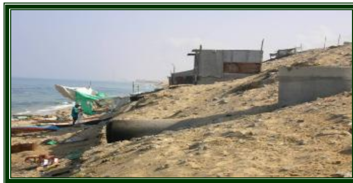
A fisherman doing his work next to waste water discharge point.
