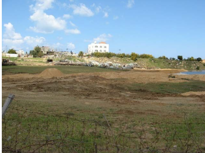
Figure 4 Emelnasser Village close to the stationery leading edge of the escaped wastewater, and the sand deposited by the CMWU contractor (Photograph by the WASH Cluster Team, Sunday 29 th March)
