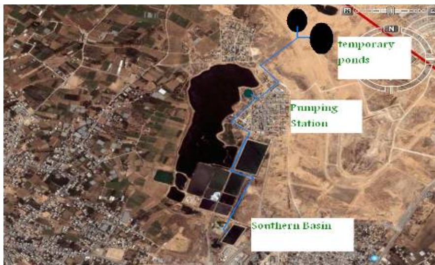
Figure 1 Aerial view of Beit Lahiya Wastewater Treatment Plant (CMWU and InfraMan 2007:8)
